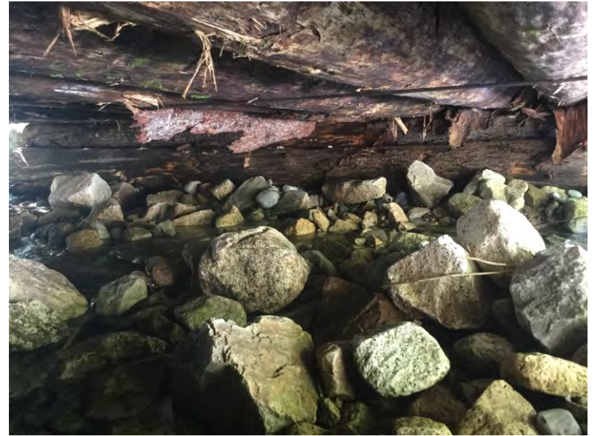
Right Bank Abutment
