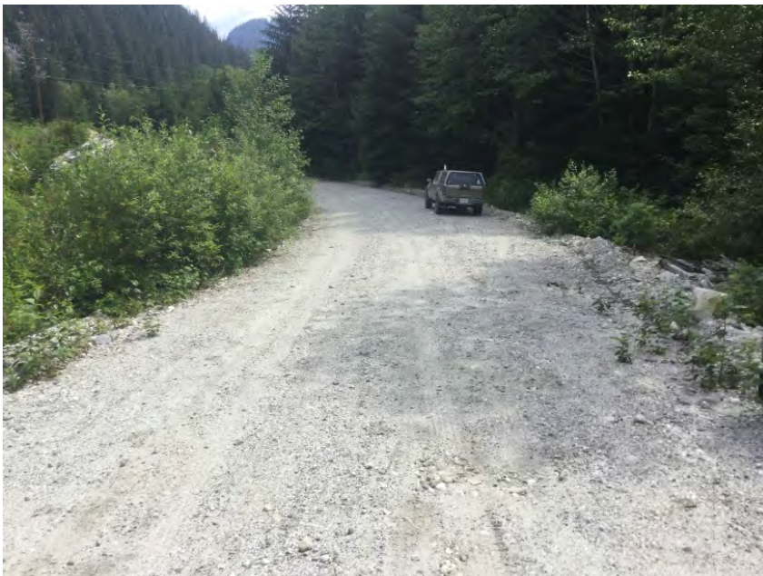
Left Approach Facing Away From Bridge
