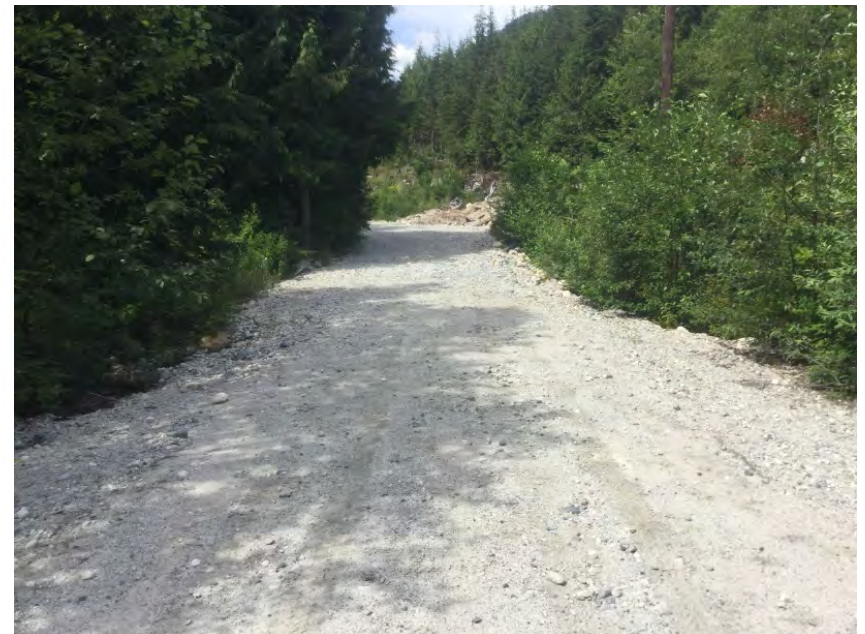
Right Approach Facing Away From Bridge
