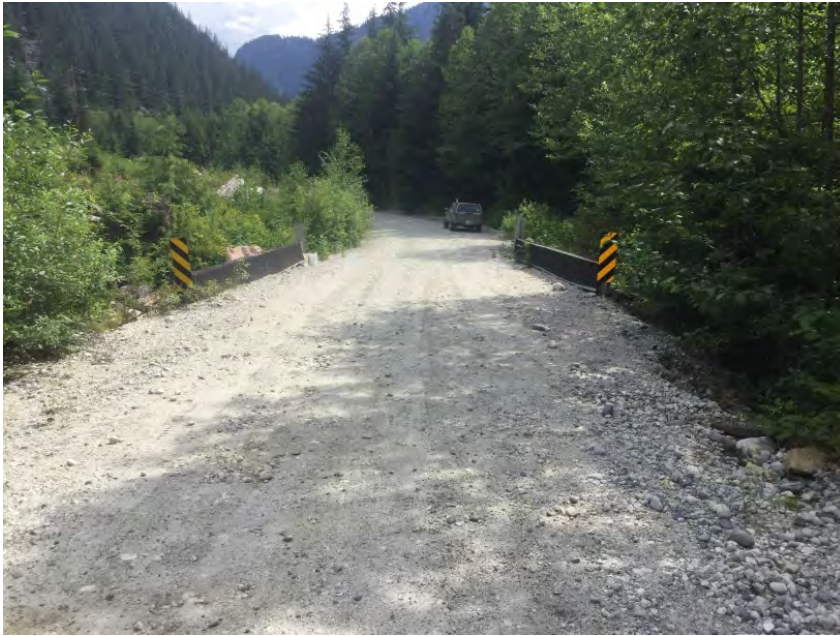
Right Approach Facing Bridge
