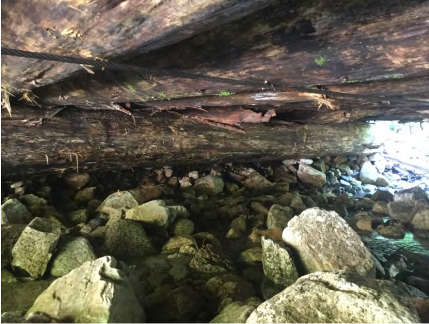
Left Bank Abutment
