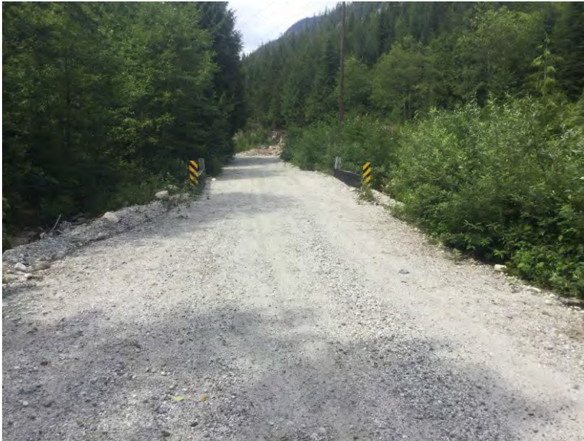
Left Approach Facing Bridge
